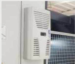
Electrical Cabinet Cooling System
